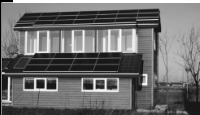
UNI-SOLAR®-US-64-modules on a holiday cottage 'De Leguaan', Netherlands.
